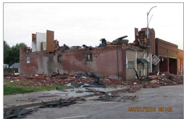
The second story of a brick building was blown off by an EF2 tornado that ripped through Mt. Olive on May 20, 2013.
